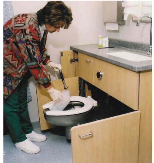
The combined lavatory/concealed water closet modules offer a convenient water source in patient rooms and serve as an efficient patient care station for medical staff.
