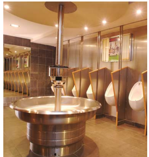
A Bradley Circular Classic Washfountain in stainless steel serves as the visual centerpiece of the men's washroom at Lloyd's No. 1, The Trafalgar. The washfountain is as economical as it is practical for the washroom's design - the unit accommodates up to eight users at one time.
