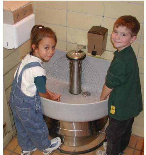
Kindergarteners are able to easily wash their hands using their new foot-controlled Bradley Terreon Classic Juvenile Height Washfountain.
