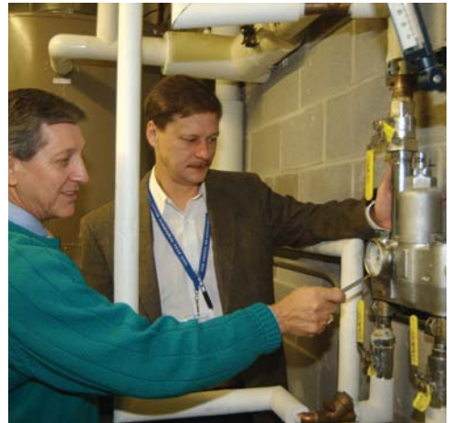
Jim Goodale with Hunt Warren (left) and Josh Robison (right) inspect the new Bradley high-low Navigator TMV.
