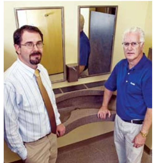
Ryan Chewning (l), with Bradley Representative Jim Volk (r), values that ndite is virtually maintenance-free, since there is no need for batteries or electricity.
