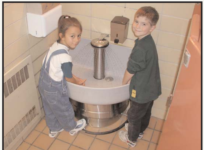
Kindergarteners are able to easily wash their hands using their new foot-controlled Bradley Terreon Classic Juvenile Height Washfountain.
