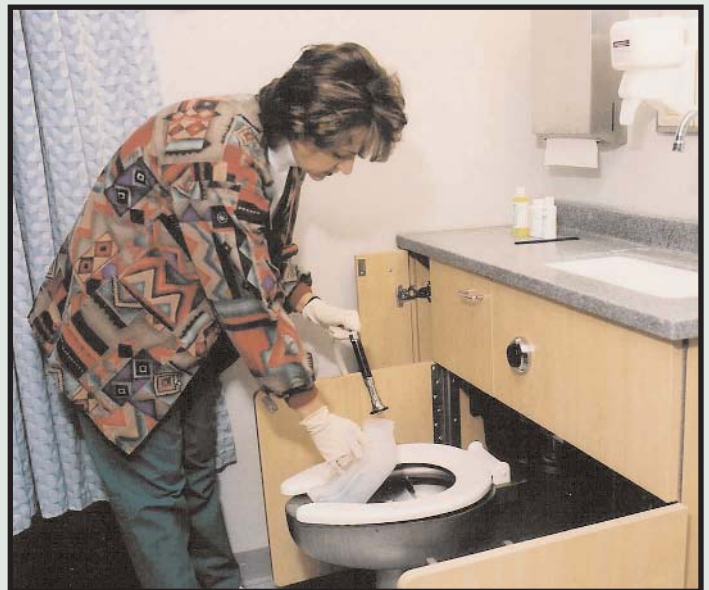
The combined lavatory/concealed water closet modules offer a convenient water source in patient rooms and serve as an efficient patient care station for medical staff.
