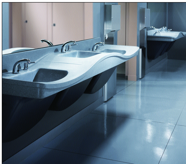
Most lavatory systems have built-in thermostatic mixing valves that are properly sized for the handwashing station.
