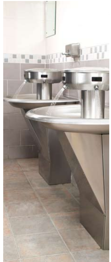
Heavy-duty stainless steel washfountains are extremely durable, and the supplies and waste valves are concealed within the pedestals.
