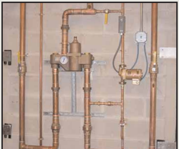
Navigator TMVs are designed to fit virtually an application, and can be easily retrofitted for an existing system like the one at NovaCare Complex.
