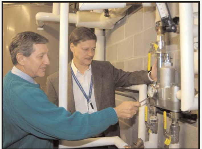
Jim Goodale with Hunt Warren (left) and Josh Robison (right) inspect the new Bradley high-low Navigator TMV.
