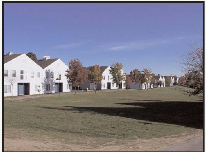
Bradley TMVs installed in the University’s seven student apartment clusters help control water temperatures and provide scald protection for students.
