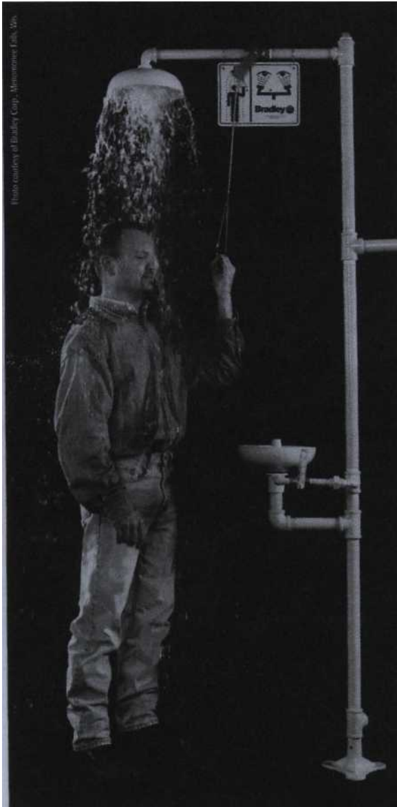
Emergency fixtures, such as this shower and eyewash unit, should be accessible within 10 seconds of hazardous workstations.
