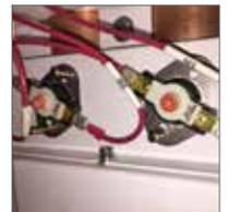
set of circuits that monitor over temperature conditions. Should overheating occur, each sector of the heat exchanger has a dedicated thermal switch that breaks power. Normal operation cannot be resumed until the safety switch is manually reset.
